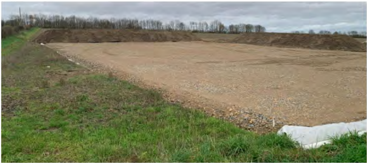
Image 17: Newly laid construction compound (Elsham Lincoln Pipeline)
