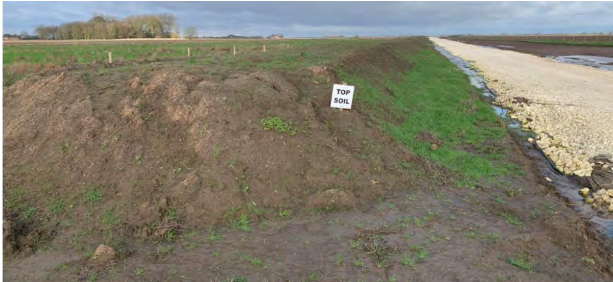
Image 16: Example of Soil Stores Next to Temporary Haul Route
