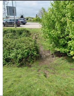
Photo B – Worn verge/embankment looking west towards A46
