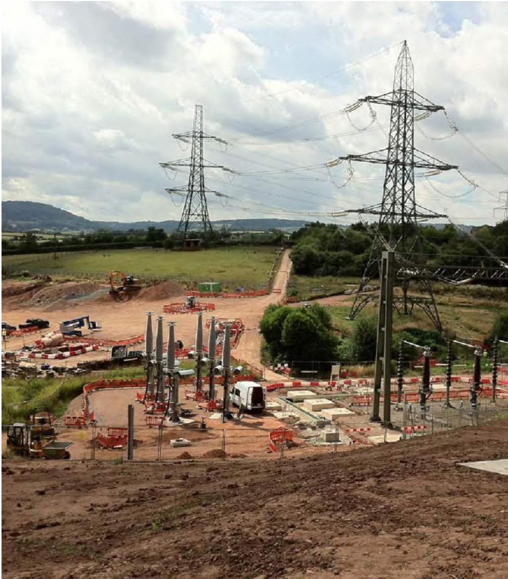
The undergrounding of electricity cables at Ross-on-Wye
