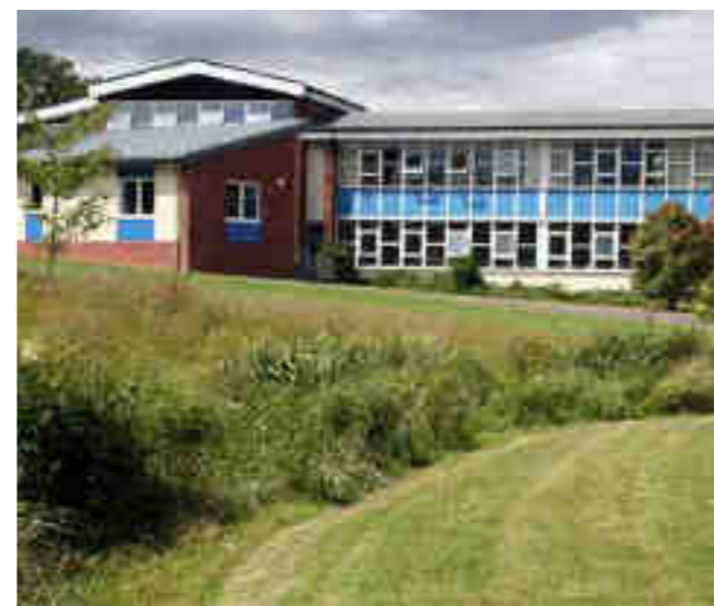
Conveyance swale at Waseley Hills High School, Worcestershire.
