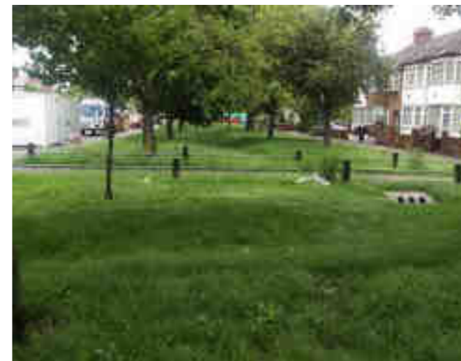
Highway runoff is intercepted using a chute gully and taken into a conveyance swale at this retrofit SuDS project. Devonshire Hill, Haringey.
