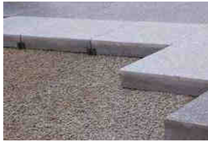
Plastic spacers are used to form open joints between standard slabs at Abbey Park Campus Leicester College, where all hard landscape areas, including the pedestrian entrance plaza to the building, are used for storage.
