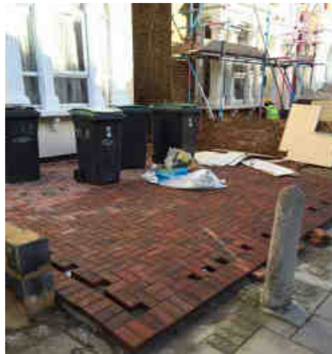
Paving over front gardens with impervious surfaces is increasingly common. This example could easily have been permeable block paved.
