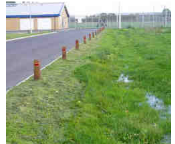
Pershore High School, Worcestershire. Low risk access road with 1.2m wide filter strip source control and conveyance swale.
