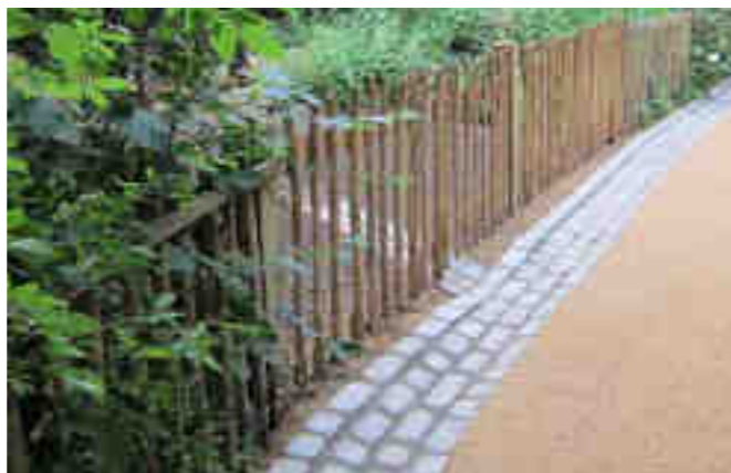
A granite sett channel collecting and conveying runoff at Holland Park, London.
