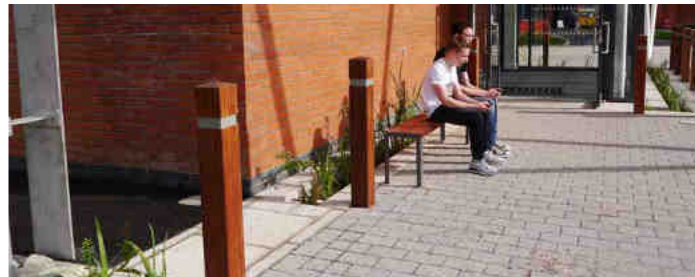
Permeable paving and planted open channels collect runoff from hard surfaces at Bewdley School, Worcestershire.
