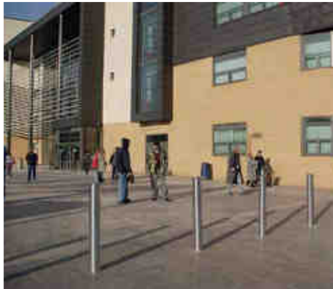
SuDS components such as permeable pavements provide interception losses. Long-term storage can also be incorporated into the pavement design and they can be used for rainwater harvesting in certain situations,
