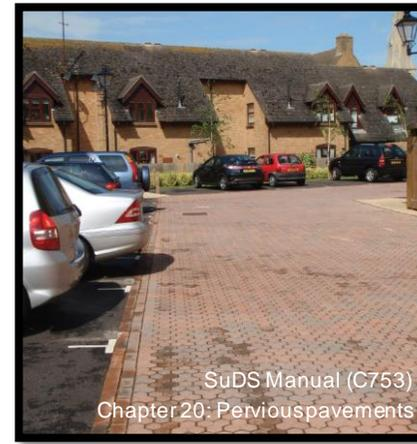
Pervious pavements can be considered in SuDS design where there is suitable infiltration and the groundwater level is low enough.
