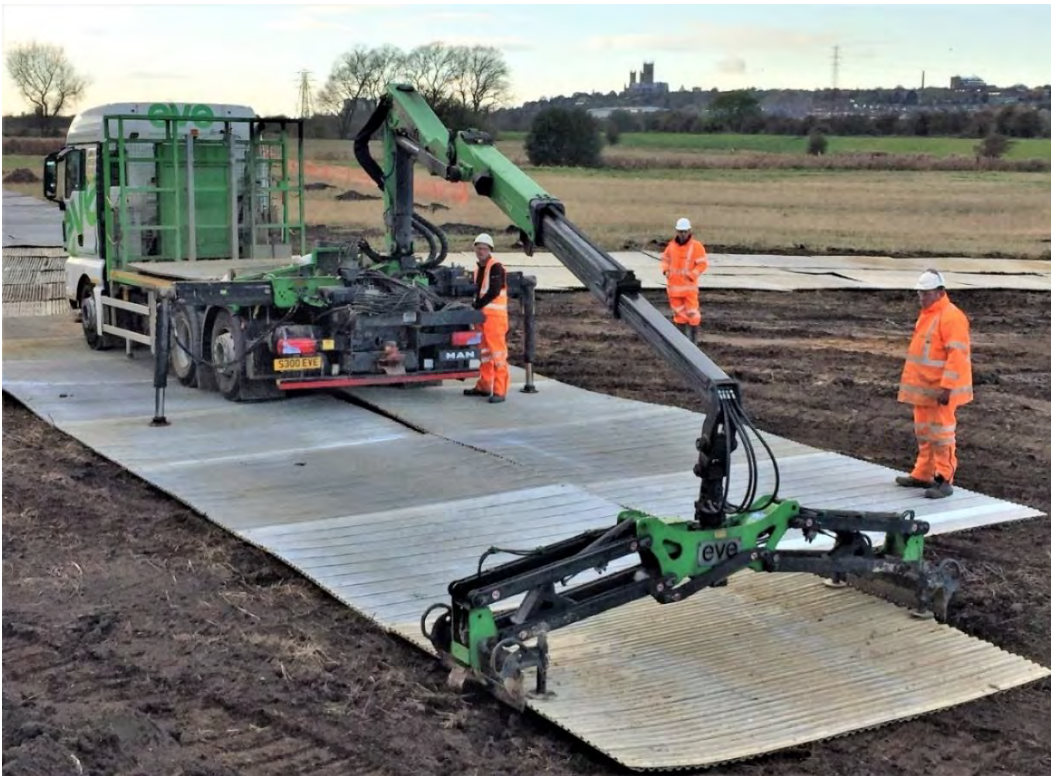
Plate 3: Laying of metal trackway close to the Witham; Cathedral in distance
