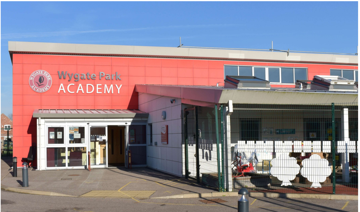
Wygate Park Academy in Spalding, funded with developer contributions
